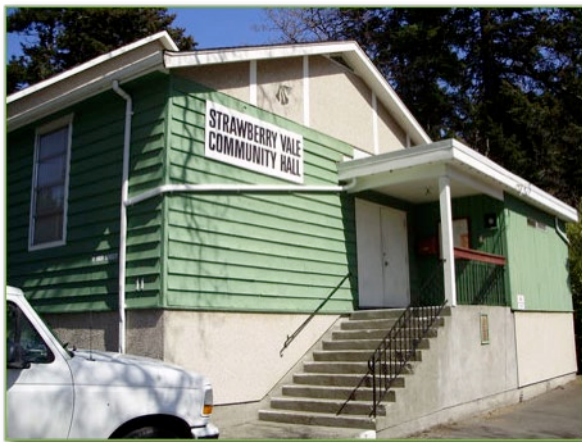
Strawberry Vale Community Hall is one of the oldest community facilities in View Royal.
