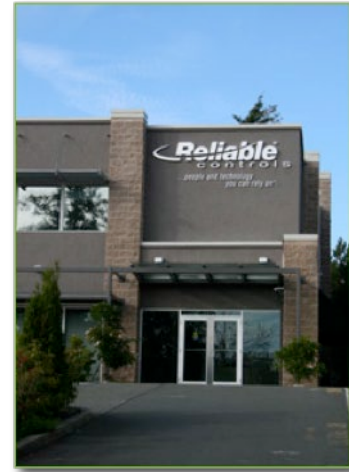
Reliable Controls – Technology development is a dynamic and evolving sector that can provide good paying jobs.
