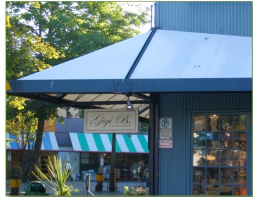
Awnings provide weather protection for sidewalks.
