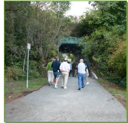
A pedestrian tunnel under the E&N rail tracks connects the Thetis Vale subdivision to the Galloping Goose Trail.
