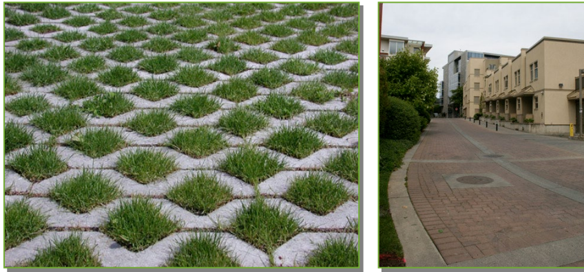
Vegetated and hard pervious ground treatments reduce stormwater runoff and promote natural filtration.
